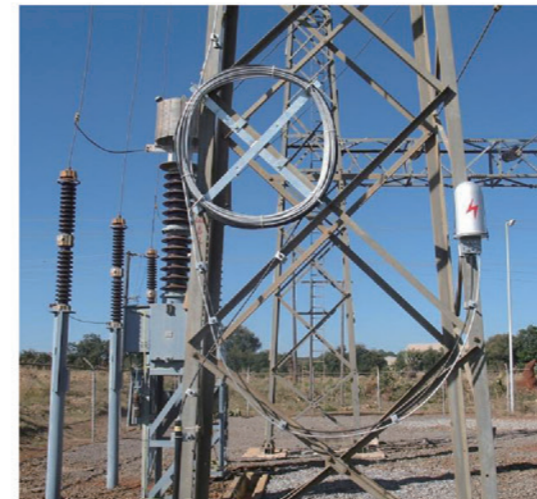
Joint box Installation
